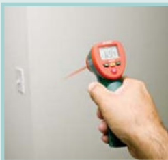
Check building for insufficient insulation
